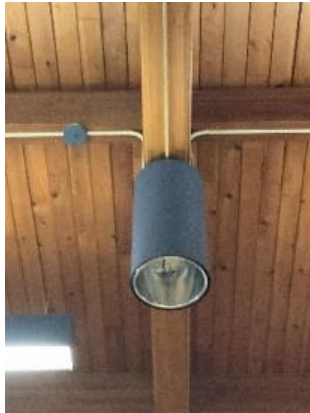
Metal halide fixtures in media center
