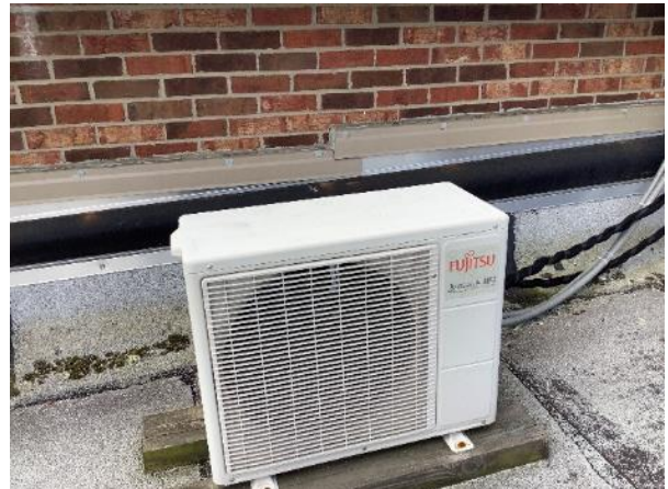
Split type heat pump outdoor unit
