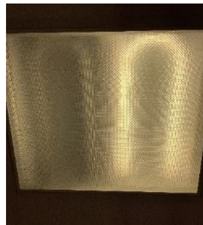
2' x 2' U-shaped T8 lamp fixture
