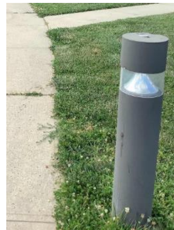
Bollard fixture with LED lamps
