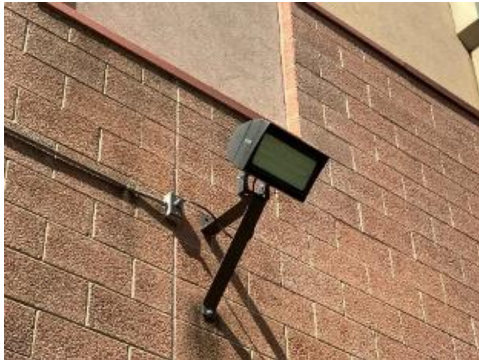
Wall-mounted LED fixture
