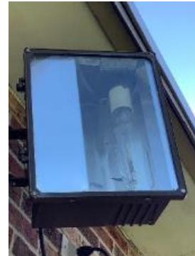
Exterior metal halide lamps
