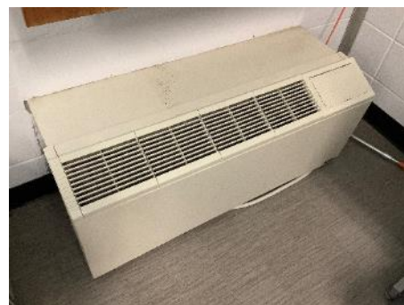
Packaged Terminal Heat Pump in main office
