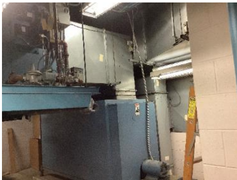
Gymnasium AHU and furnace
