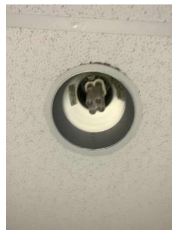
Recessed can fixture with CFL
